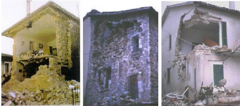
**Fig. 1.2.1.** First damage mode: collapse mechanisms [3]
