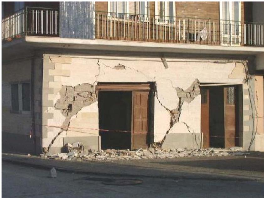
**Fig. 1.1.2.** Diagonal shear cracks [2]
