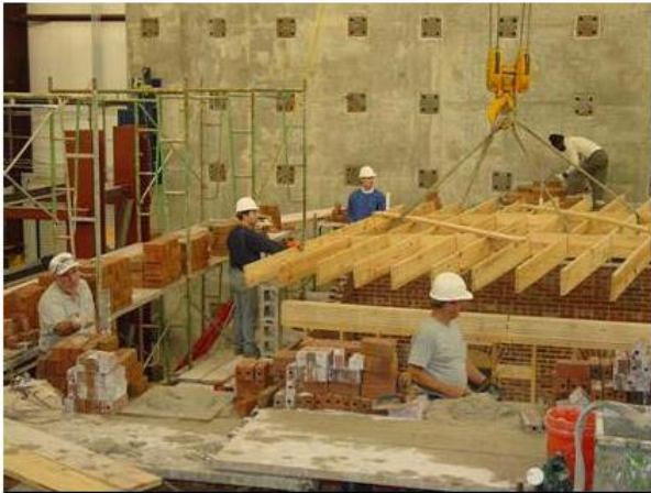
Figure 6.17. Assembly of the floor systems
