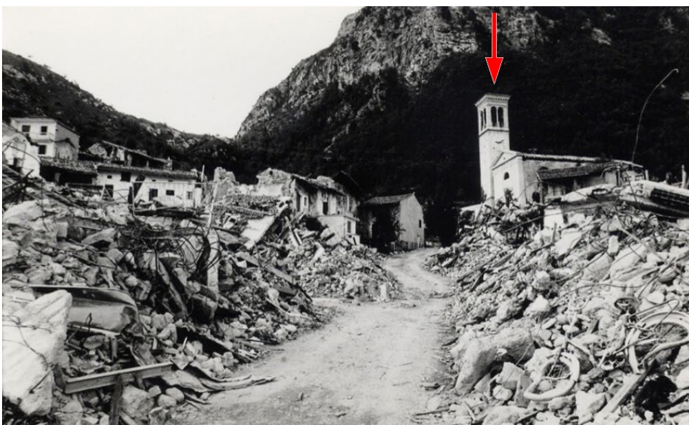
Figure 15. Seismic damage in Friuli (1976). A bell tower unaffected by disaggregation is highlighted.
