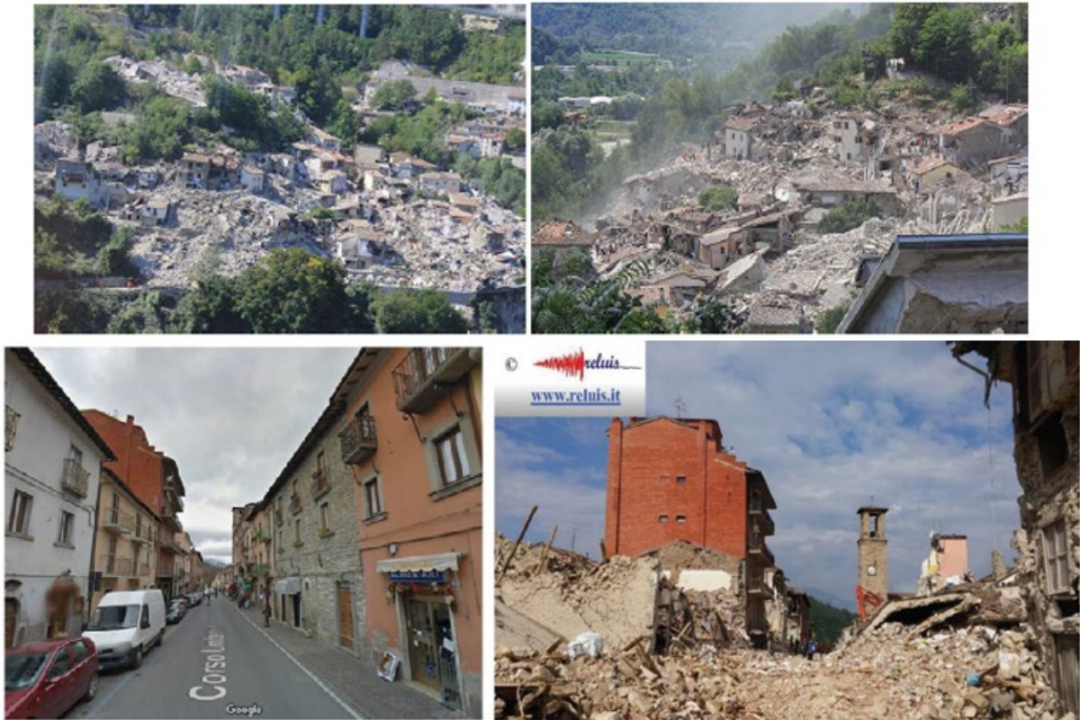
Figure 1. Disaggregative effects caused by the seismic events in Central Italy, 2016 [1]. Top: Pescara del Tronto. Bottom: Corso Umberto I in Amatrice before the event (left) and after the event (right).
