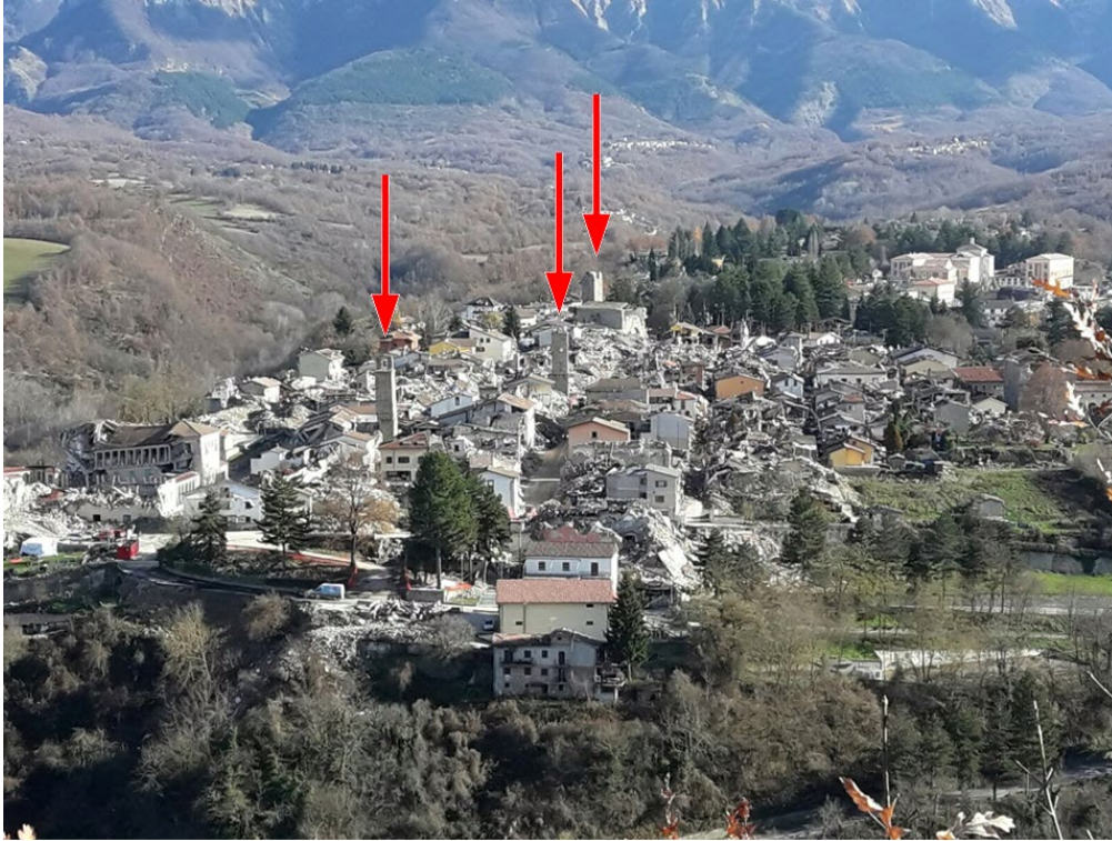
Figure 14. Seismic damage in Amatrice (2016). Masonry towers that were unaffected by the widespread disaggregation are highlighted.
