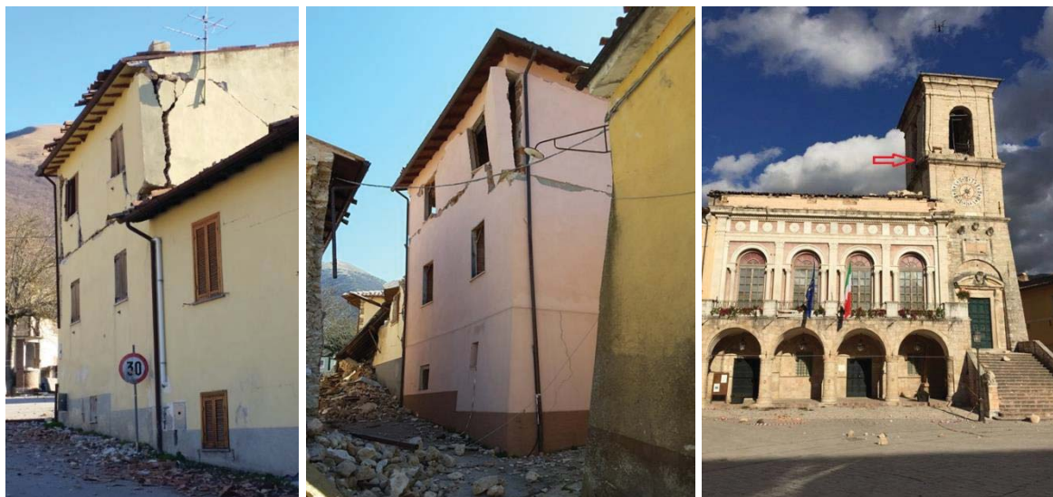
Figure 5. Pure shear failures (courtesy of Alessandro De Maria)
